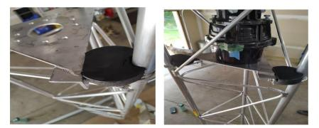
I now needed a tube extension to be able to connect the 6-foot mast to the rotor now installed in the second section. I purchased from Lowe's an 8-foot steel fence post which I used as a center shaft extension. I inserted the 6-foot mast inside the fence post and drove two screws in a "cross" pattern to hold them together.
